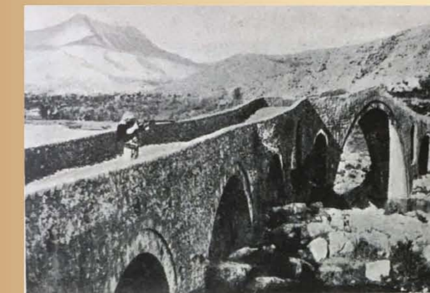
An Eleven-Span Greek Bridge, 500 years old.
